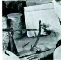
Checking the "bend value" of wire is highly important for uniformity.
