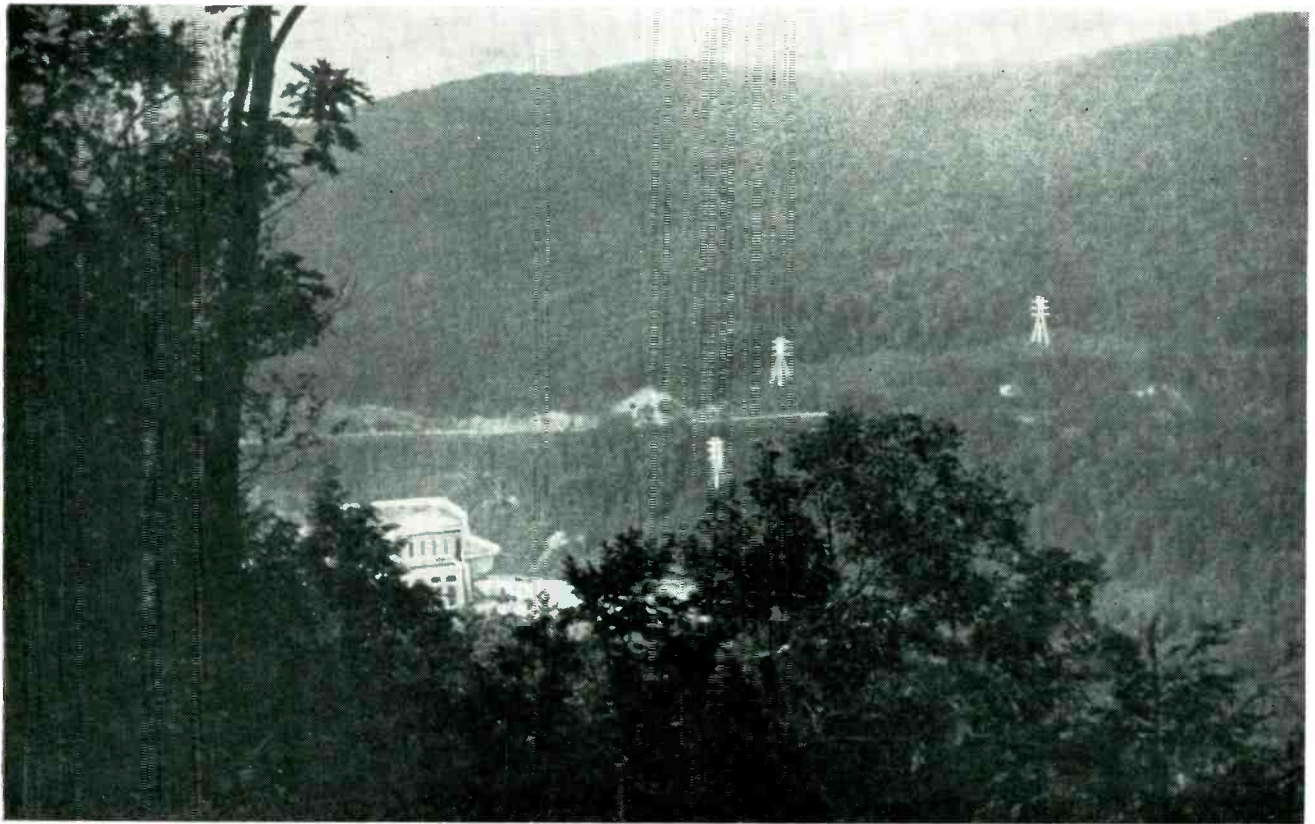
View of West hydro electric station, taken from reflector location atop Hunt's Mountain, shows clear path for reflected 960-megacycle signals transmitted at Stewart's Bridge. Path shown corresponds to ½-mile leg illustrated in plan drawing below
